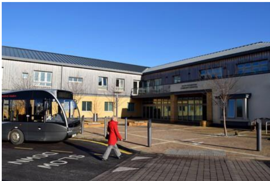
South Petherton Hospital
