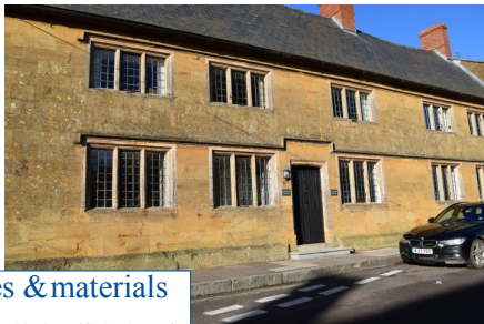
Ham stone, slate roof, mullion windows
